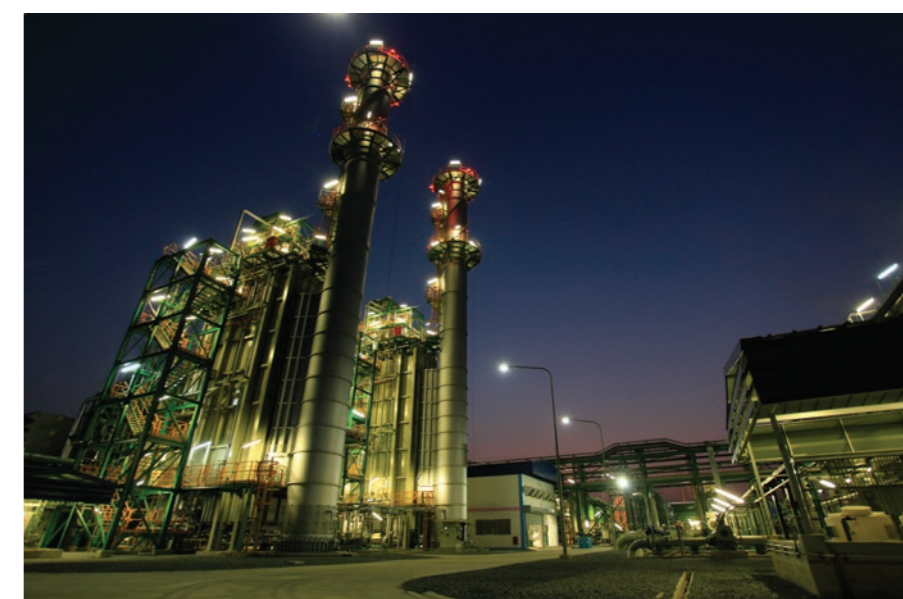
Johnson Controls YD Chillers provide the cooling capacity to meet the GTIAC requirements of Navanakorn Electric Co. Ltd. CCGT Cogen Plant, Thailand.
